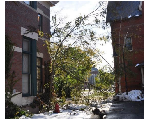
Fig. 11 Damage caused by the “Snowtober” Storm, October 2013
