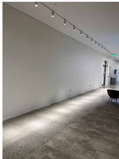
2 View of the wall from the Elevator
